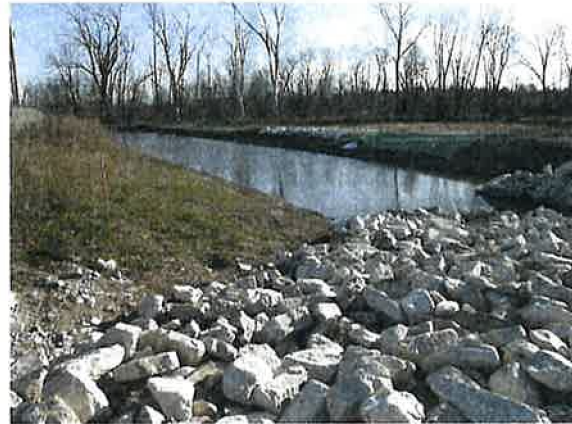
Wet Bottom Detention Basin – Orientation Northeast
