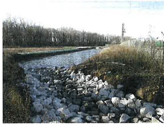
Wet Bottom Detention Basin – Orientation Southwest
