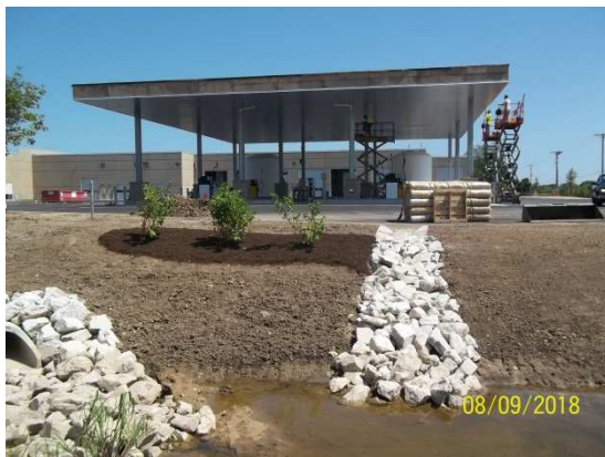
RipRap Parking Lot Drainage
