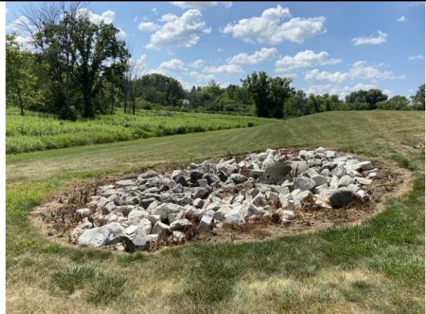
Pond 2 primary outfall into wetland area
