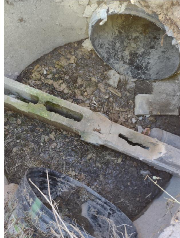
Inside of outlet structure. Water from the pond drains through the primary outlet pipe, through the 4" dia hole in the block wall inside the structure then discharges out the secondary outlet pipe.
