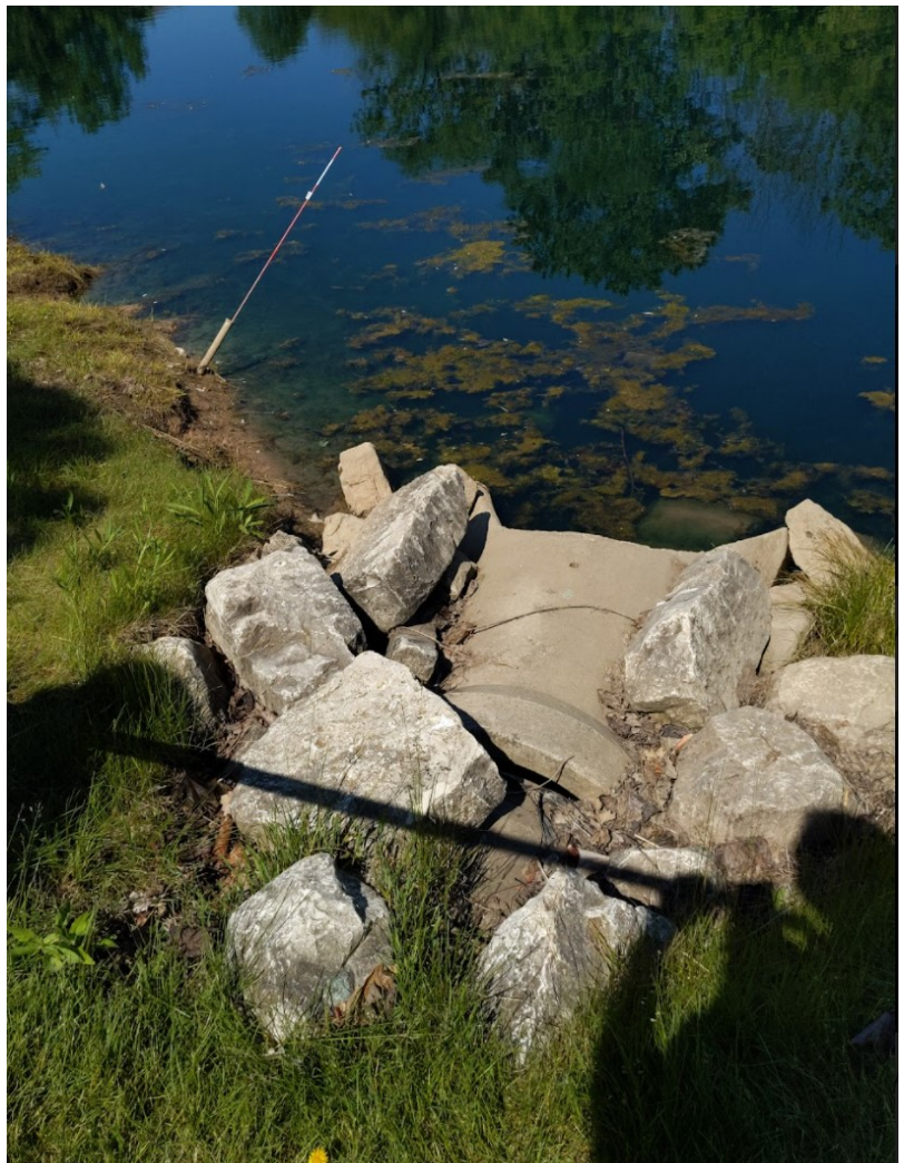
South infall pipe that is broken off at the endwall section.
