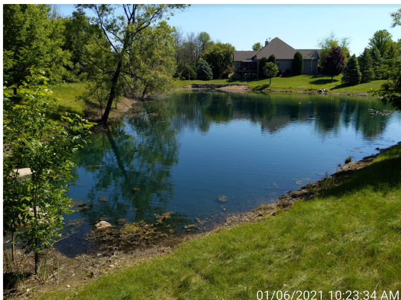
View of overall wet pond. Trees and woody vegetation shown here that should be removed.
