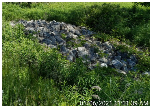
View of emergency overflow weir.
