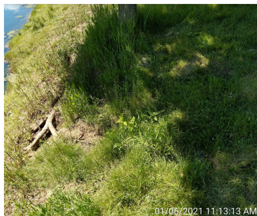
View of exposed roots and erosion.
