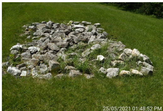
Emergency riprap outflow weir
