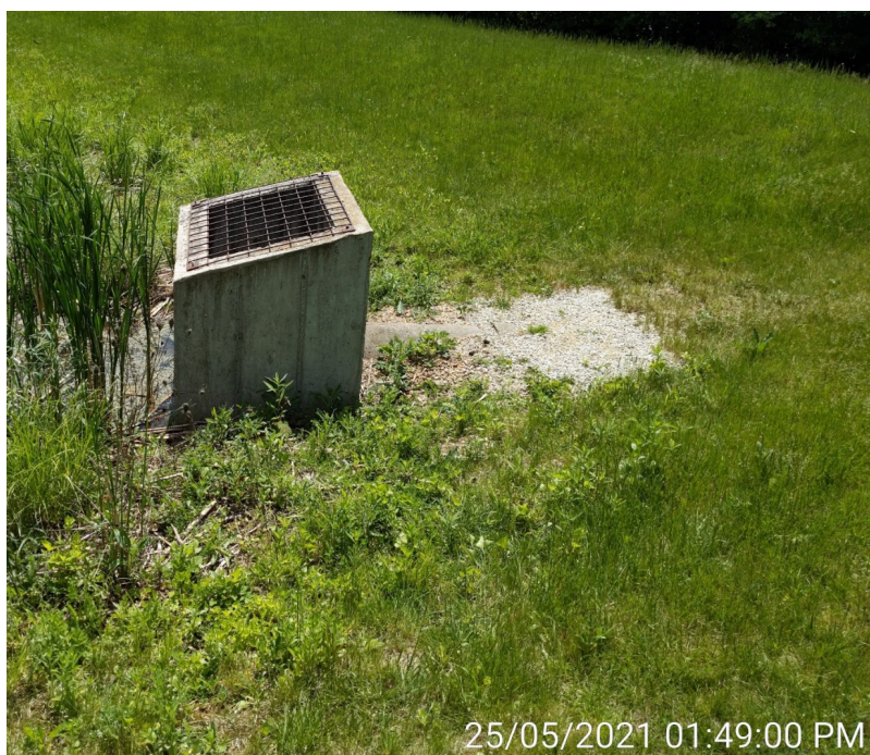
Outlet structure. Outlet pipe is exposed. When infall pipe sediment is removed for riprap outfall, excavated material can be placed here to cover pipe.
