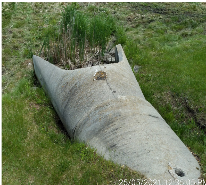
Outlet pipe with broken off endwall section
