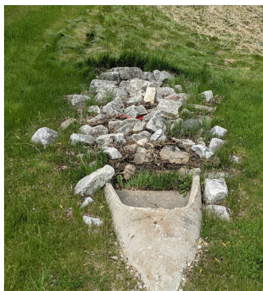
Infall at southeast corner with sediment in riprap outfall
