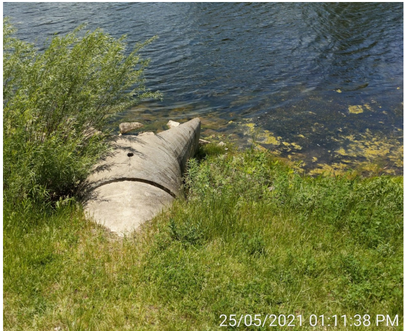
Infall pipe from Dry Pond #3 with detached end section
