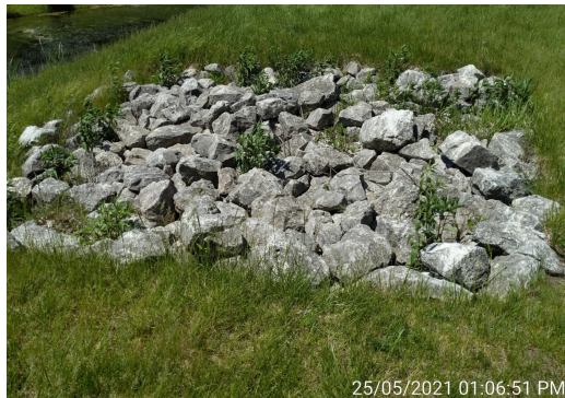
Emergency riprap outflow weir
