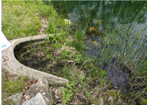
Infall pipe at south edge, showing sediment
