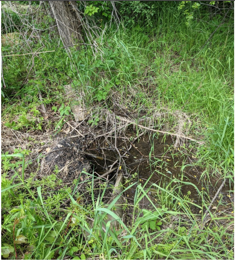
View of outlet pipe in the wooded area, water flow is being hindered by sediment and vegetation
