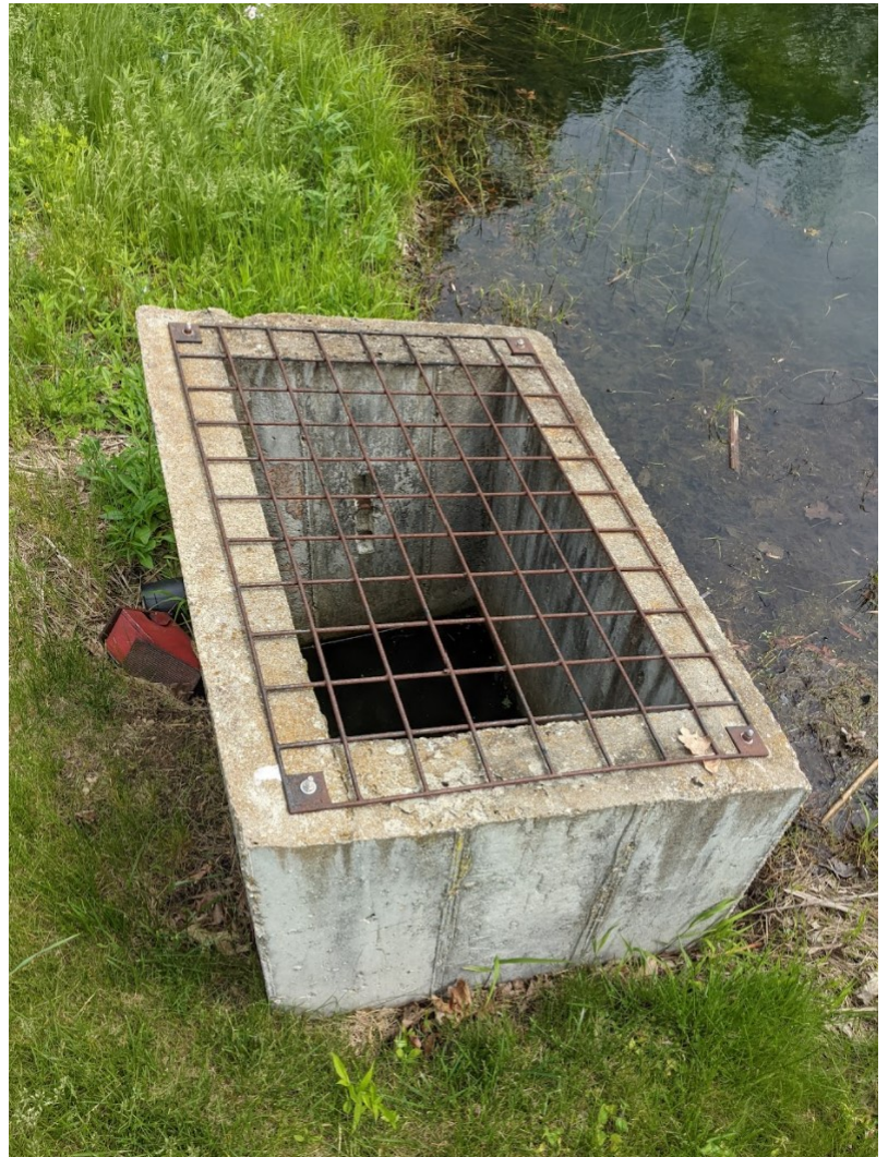
Outlet structure with rebar grate bolted down
