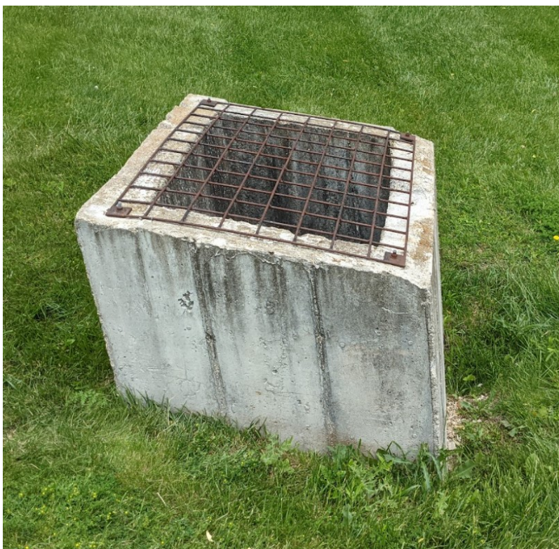
Outlet structure with rebar grate bolted down
