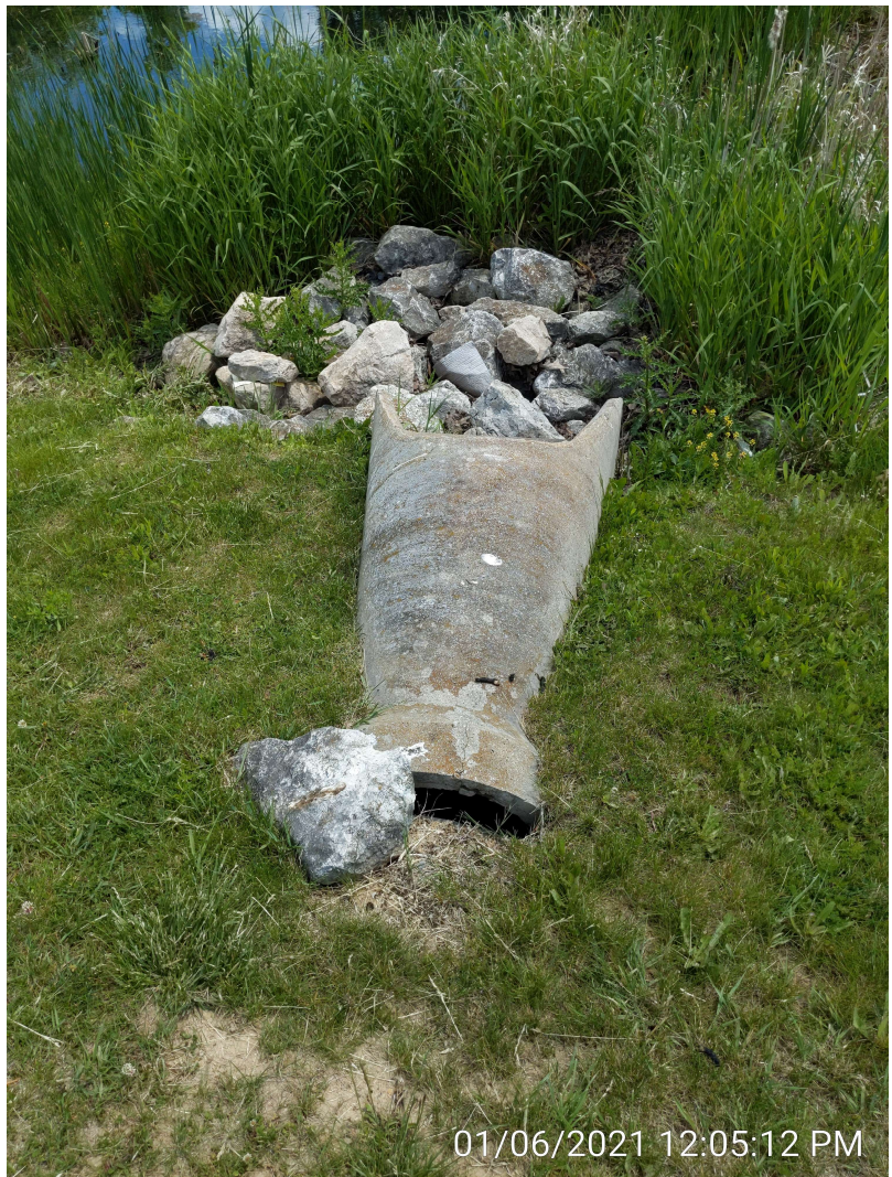
Endwall at southwest corner that is breaking off
