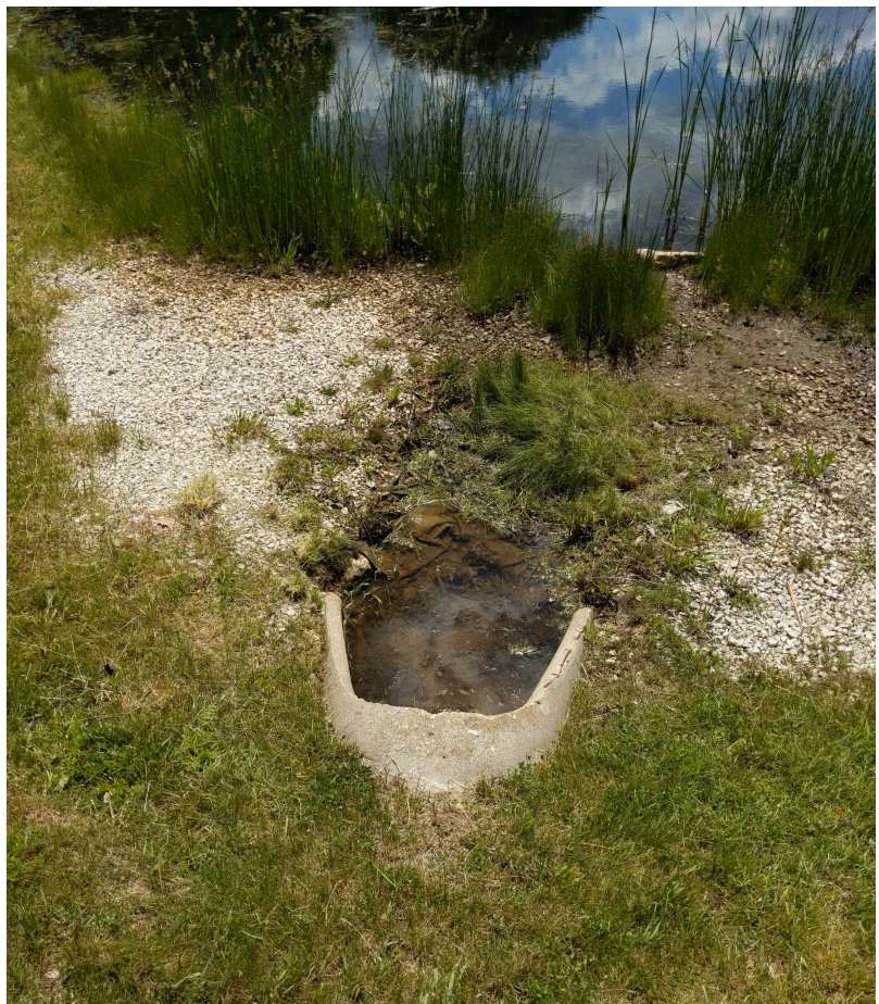
Endwall at southwest corner that is breaking off
