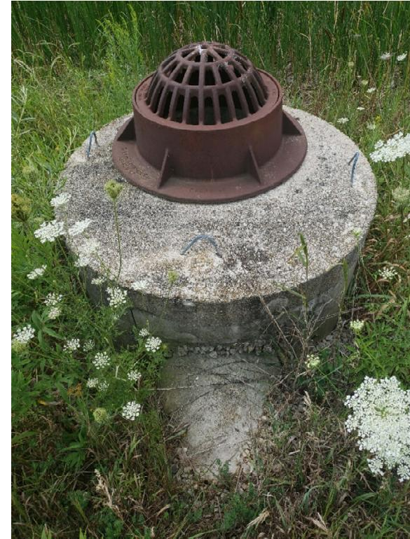
Casting and primary outlet pipe out of outlet structure.
