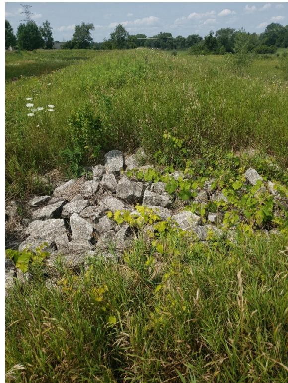
Riprap in emergency spillway along the north side of the pond berm.
