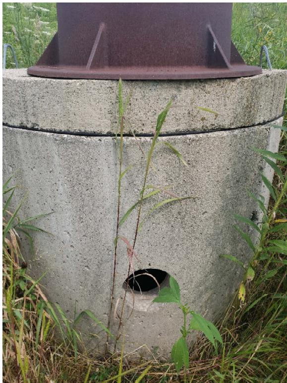
7" hole in pond outlet structure.
