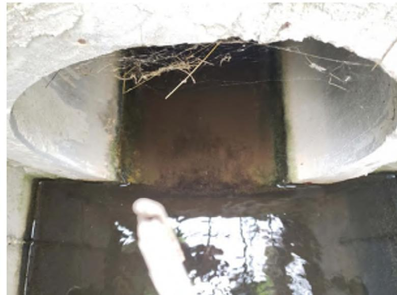
24" rcp pipe out of the pond outlet structure. Some sediment build up in the structures sump that needs to be removed.
