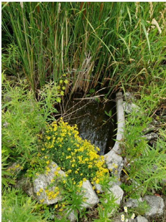
Outlet structure downstream endwall. 24" rcp pipe. Vegetation in front of structure needs to be removed.
