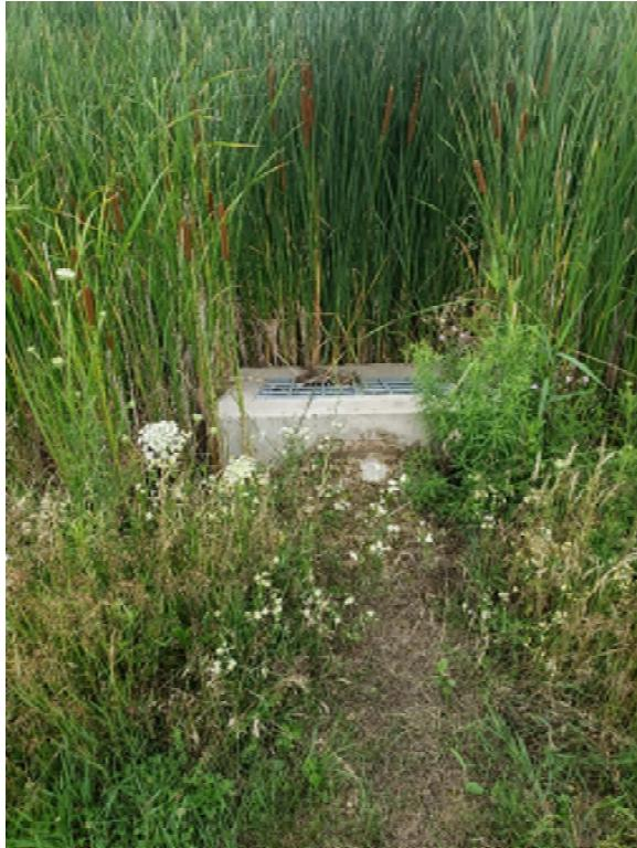
24" x 36" pond outlet structure. Maintenance required to remove vegetation in front of structure and remove nest on top of grate.
