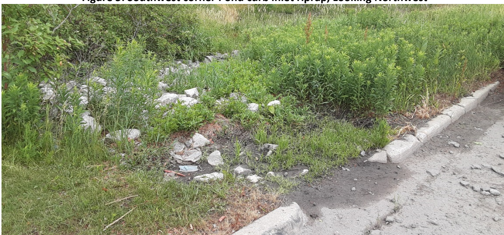
Figure 6: Southwest corner Pond curb inlet riprap, Looking Northwest
