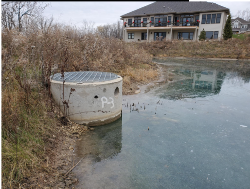
Figure 2: Pond 3 Outlet Structure
