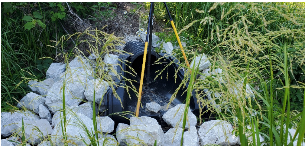
Figure 6: 15" HDPE Pond Outfall, Looking North
