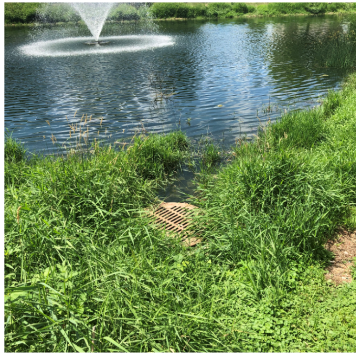
Outlet Control Structure
