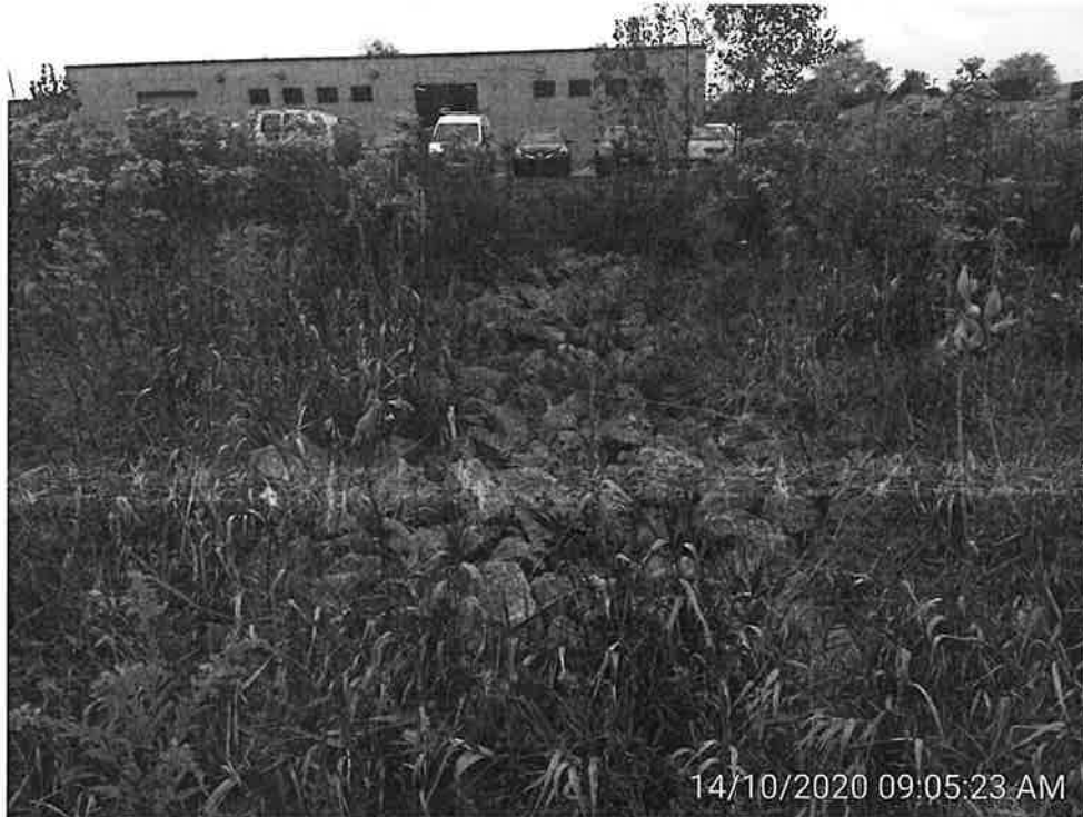
Photo #3: Emergency Spillway
