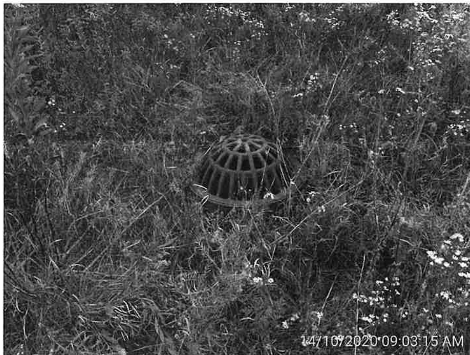
Photo #2: Outlet structure/stand pipe
