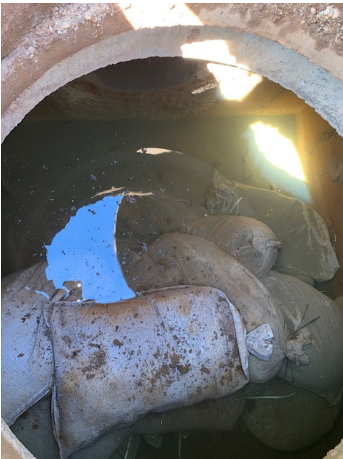
Storage Chamber - Sand Filter
