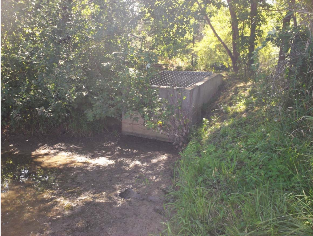
Photo 3: Outlet structure front intake silted.
