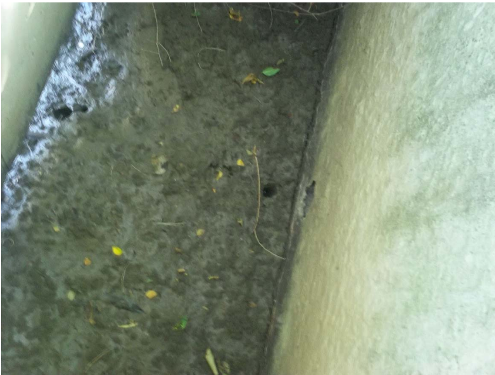
Photo 4: Outlet structure bottom silted.
