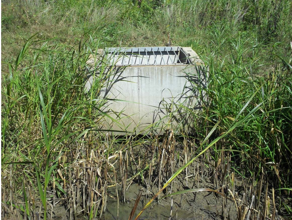
Photo 3: Outlet structure front intake silted.
