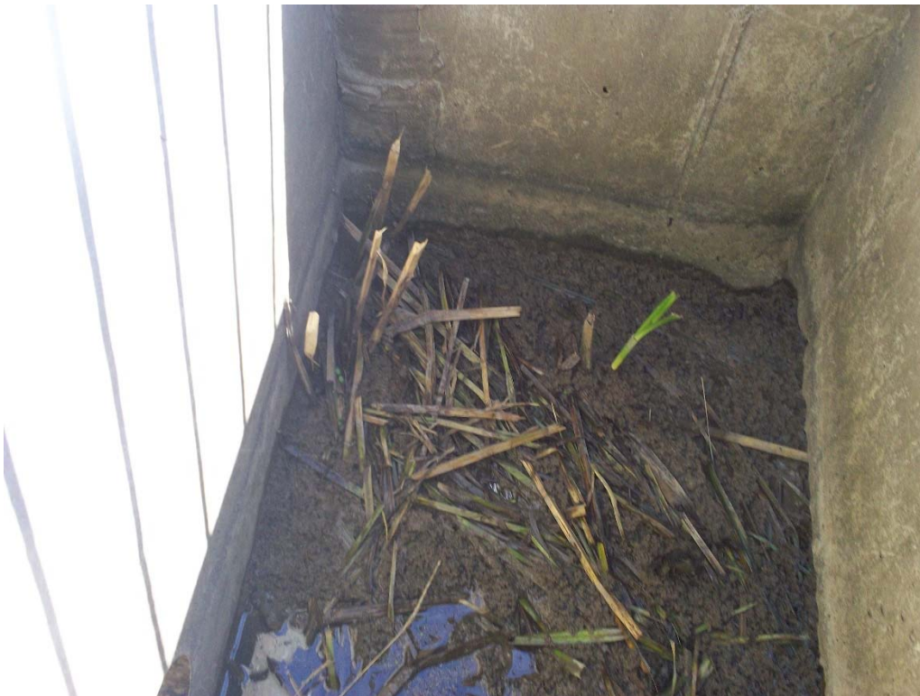
Photo 4: Outlet structure bottom silted.
