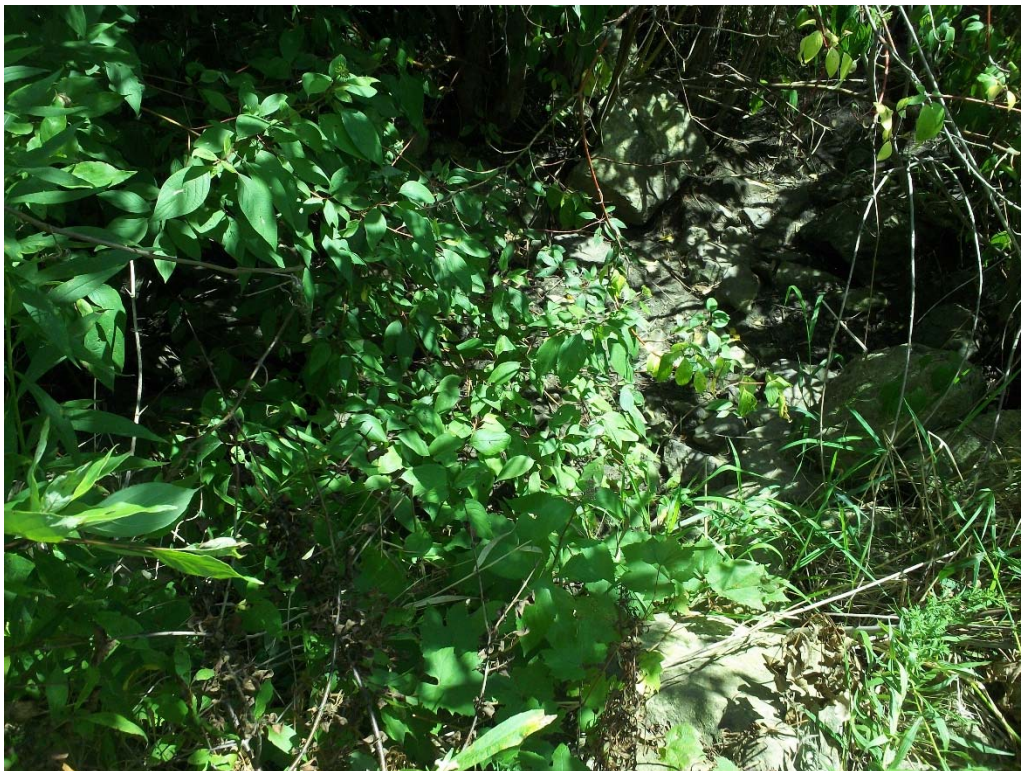
Photo 8: Outlet structure discharge pipe in wooded area.
