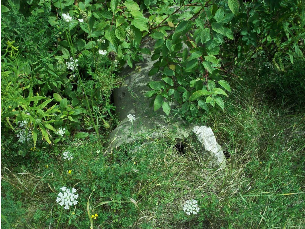
Photo 3: Outfall 1 (ES-10) heavy vegetation.
