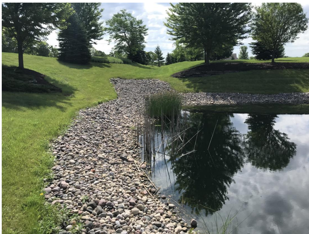
Figure 6: At northeast portion of pond; looking easterly (emergence spillway)
