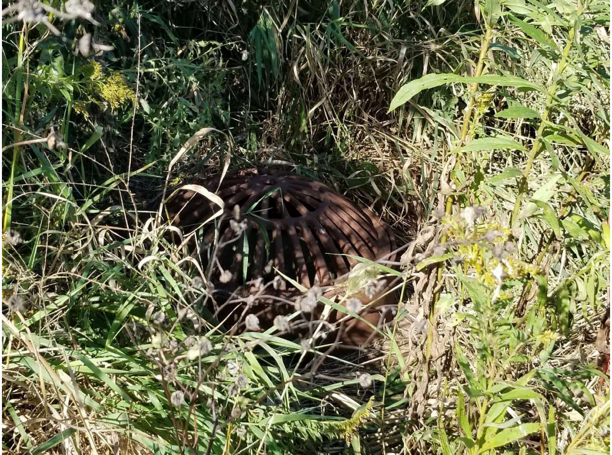
Beehive grate – outlet structure
