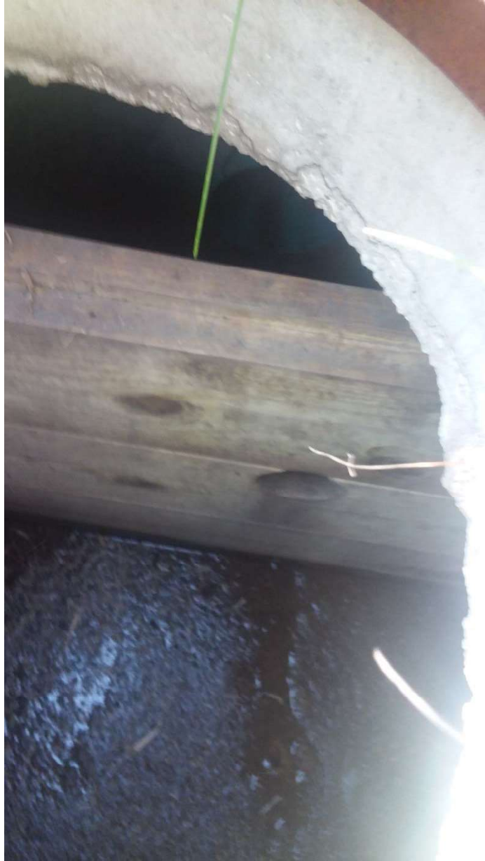
Outlet structure with baffle wall – SWP13S026
