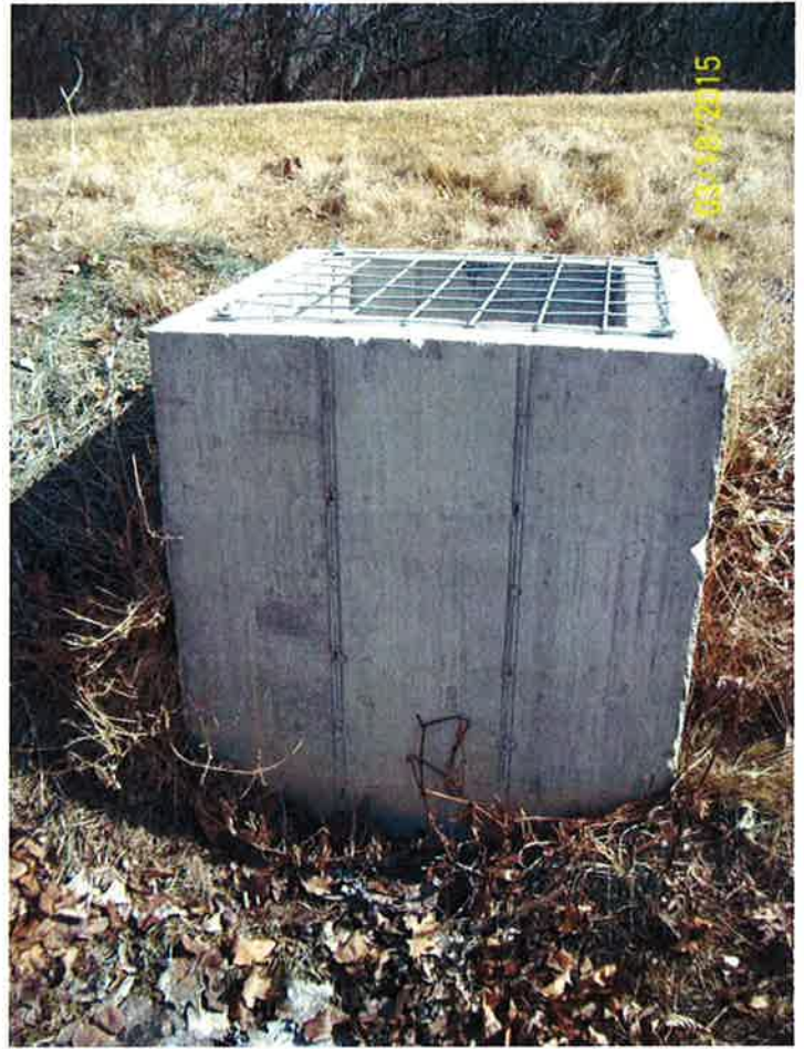
Overflow Structure ST013440
