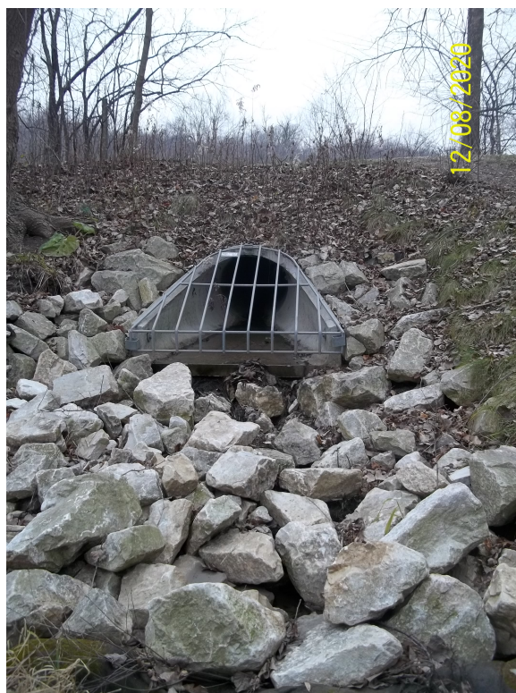
Overflow Outlet ST014269
