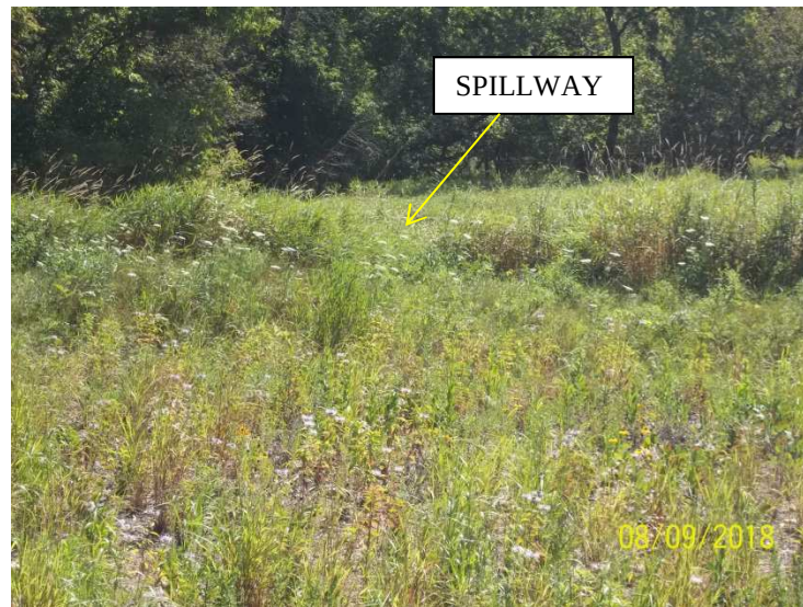
Spillway (NE Corner)
