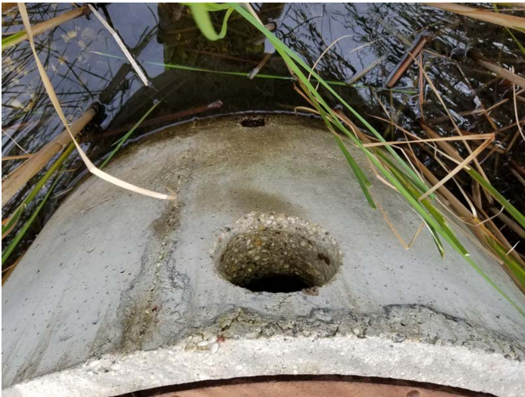
View of upper and lower orifice at control structure (from above).
