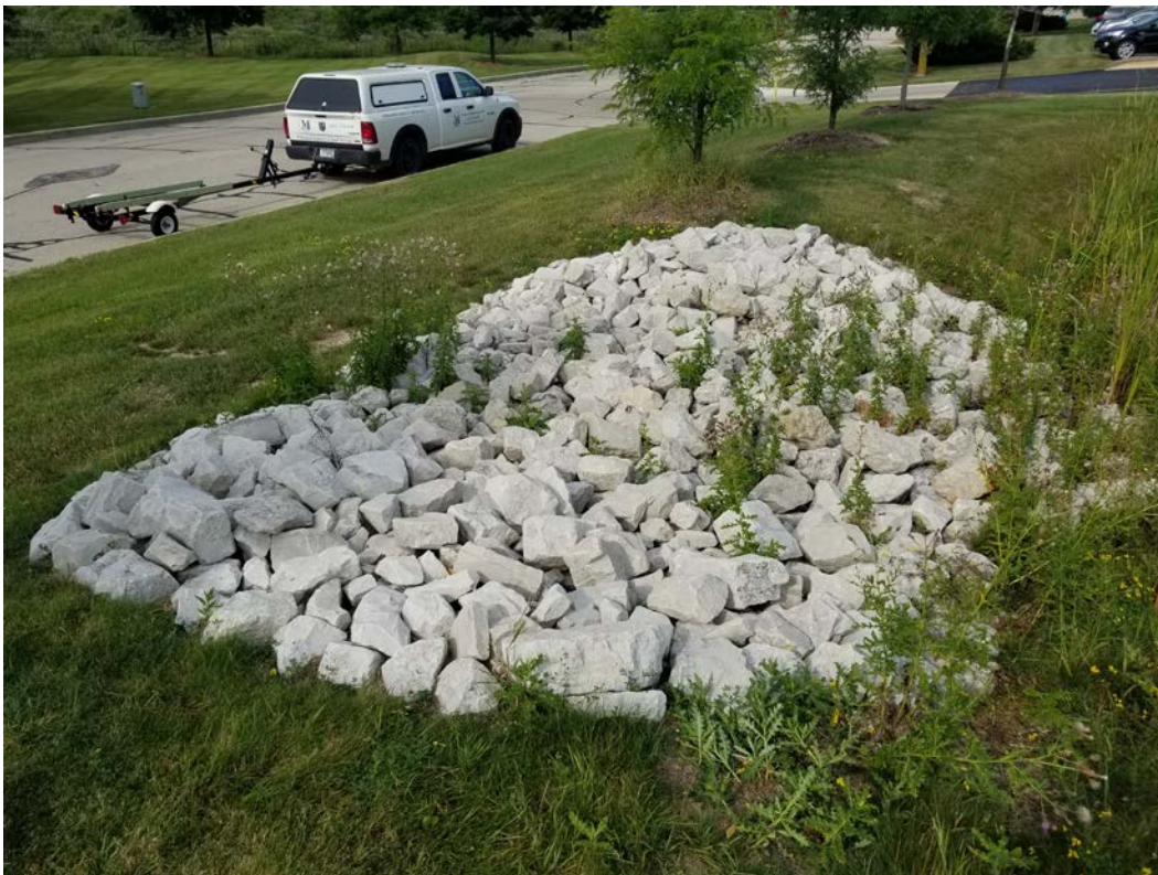
View of overflow spillway. Note minor weed encroachment into spillway. Trees on downstream side of berms are visible in the background.
