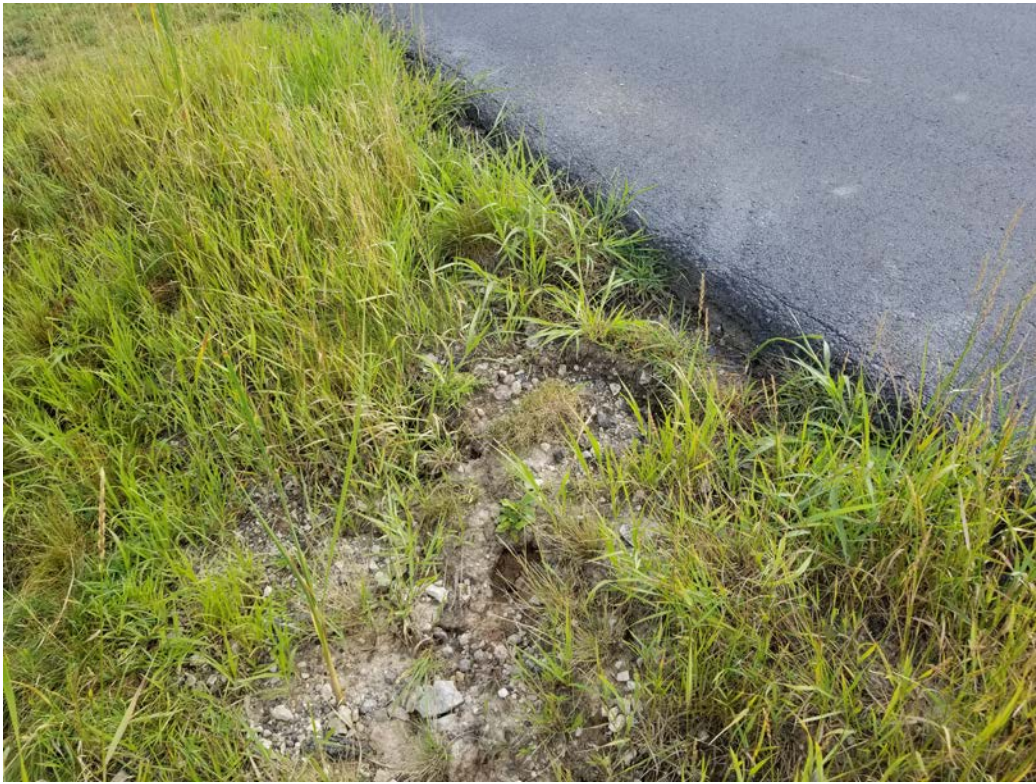
Minor erosion at edge of asphalt pavement adjacent to the pond east side.
