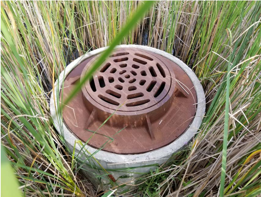
View of top of outlet control structure with Neenah casting.
