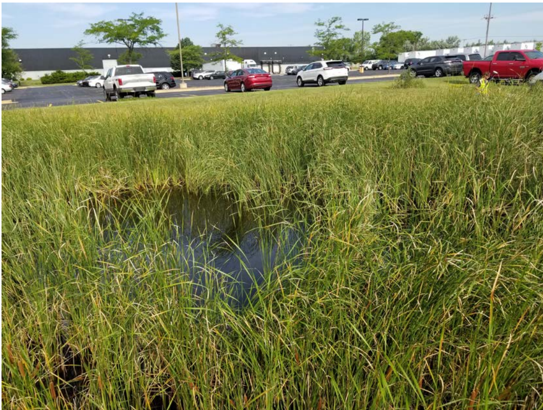
View of pond. Cattails have encroached onto all but the deepest areas of the pond. Pond depth at the center is 5 feet as designed.
