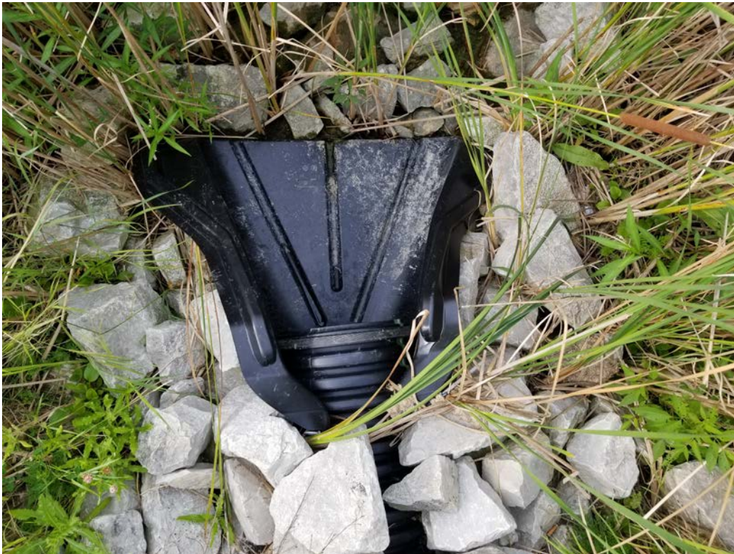
Pond inlet at NE corner. Pipe and riprap in good condition.
